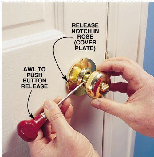
REMOVE the inside doorknob by locating the button (like our model), metal tab or wire clip on the side of the knob that acts as a release. Using an awl or small screwdriver, push the button in all the way—and at the same time—pull off the handle. Remove the door rose by inserting a small screwdriver into the small notch in the rose and twisting the tool to pop it off. Be careful so you don't chip any door paint.
