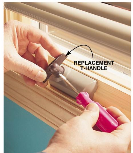
INSTALL the T-crank handle and tighten the set screw. Open the window by turning the handle counterclockwise. With the T-crank handle, window miniblinds will hang freely all the way to the windowsill.
