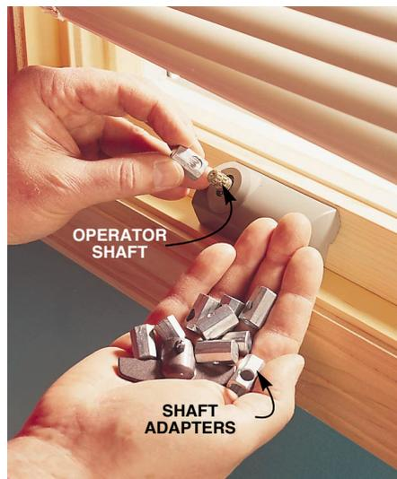
SELECT the T-handle adapter that fits tightly over the shaft of your window opener. A generic replacement handle kit comes with multiple adapters sure to fit your opener's particular shaft profile and size.
