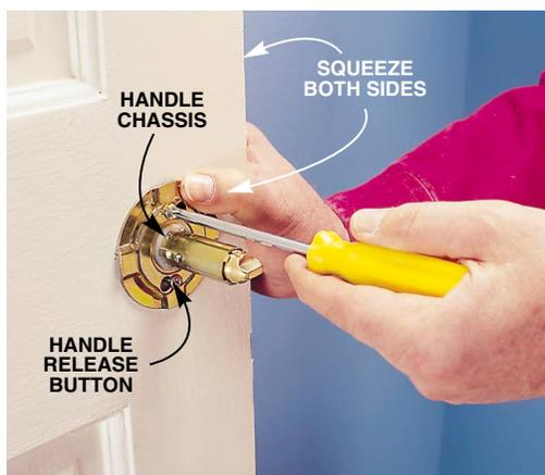
TIGHTEN the door hardware by opening the door, squeezing both sides of the assembly together and tightening the two screws on the chassis. To reassemble, snap the rose back on the chassis, depress the release button and slide the knob back on until the button pops through the hole.
